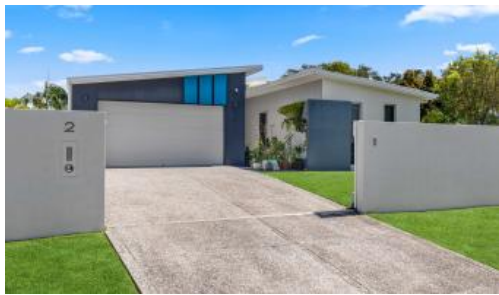
2 Wilshire Place, Pelican Waters
