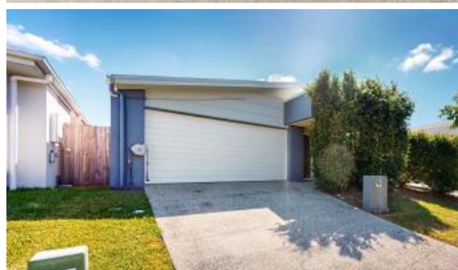
57 Burnet Circuit, Baringa
